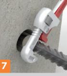
Set the rebar in the correct position and use a wrench to tighten the lock nut.
