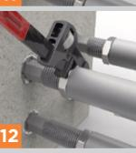
Tighten the lock nuts with a wrench.
