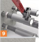
Use a wrench to tighten the couplers onto their matching rebars.
