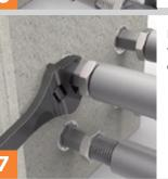
Rotate each stud with a wrench to find the correct engagement position.
