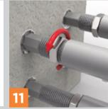
Rotate the lock nuts towards the fixed couplers.
