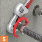
**Fix the Coupler and Secure the Splice** Use a wrench to tighten the coupler.
