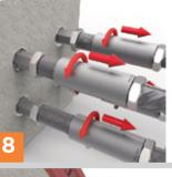
Rotate the couplers until they have reached the end of the threaded rebars.
