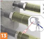
When the installation is completed check the mark on the studs as they must be inside the splicing (not visible outside the couplers).
