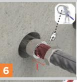
Check the distance "I" between the coupler and lock nut (still engaged at the bottom of the long thread) it has to fall between the limits indicated in table 5 below.
